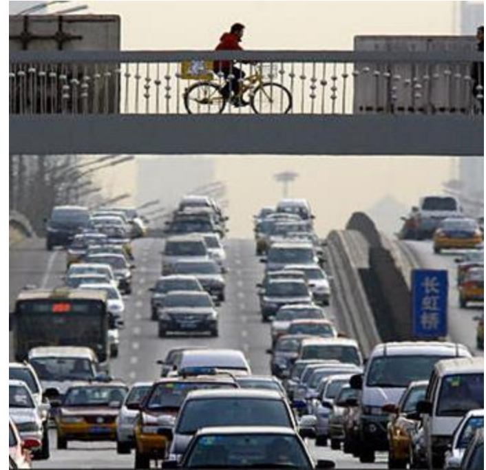
Pedestrian Walkway Bridges in Beijing, China
