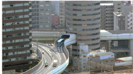
Beltway Between Commerce Layers
