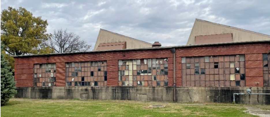
Photos: Project Site, Hangar 4 at the former Chanute Air Force Base in Rantoul, Illinois.
