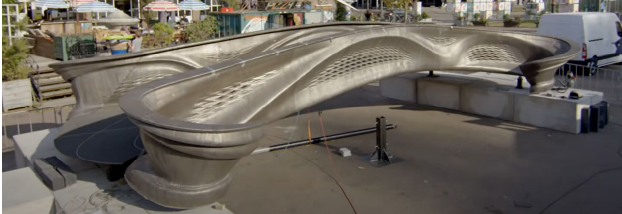
3Dprinted steel bridge in Amsterdam, by Van Wijnen and Max3D.
